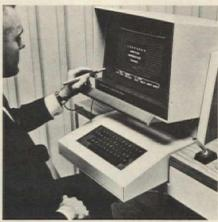
Mayo Clinic will use Lockheed's Video Matrix computer terminal, which consists of video screen, keyboard, printer, and electronic light pen. Magnetically coded card inserted in console identifies doctor as an authorized user; with light pen, doctor indicates type of treatment desired for any of his patients.
