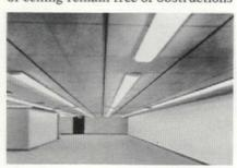
and conventional air diffusers. Our vent splines were used since they eliminated almost all branch duct work, yet provided 2½ cfm of air at almost 30 fpm without draft.
