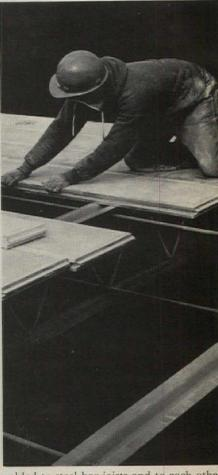
Steel-edged gypsum planks are welded to steel bar joists and to each other.
