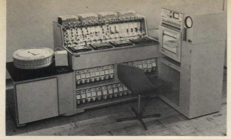
The SMA 12/60, one form of AutoAnalyzer manufactured by Technicon Corporation, automatically performs 12 chemical analyses simultaneously on a single blood sample. Automation in the laboratory means smaller chance of error in tests or lab reports. Hospitals using the AutoAnalyzer report that, since tests are performed that would not be ordered if work were to be performed by hand, the machine frequently detects incipient diseases that have no obvious symptoms.
