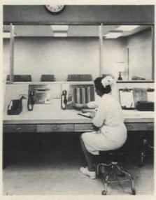
Central control station for nurse-patient communication can also monitor all aspects of patients' conditions. Executone's system will monitor arterial pressure, electroencephalogram, pulse, respiration, body temperature, electrocardiagram.
