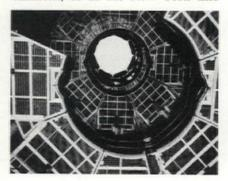
Building, few know that our knowledge of lightweight structures was applied to the construction of Titan missile silos. In these, accurate fabrication of the swingable grating platforms was essential to the smooth working of this massive assembly.
