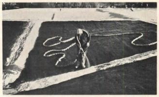
Good resistance of rigid urethane to thermal stress was critical factor in sealing expansion joints between parabolic shell sections on roof.
