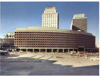
8-story One Center Plaza, Boston, which is being built in three phases (three 300-ft sections). Steel framing was chosen for the ease with which it can be expanded laterally, and for the interior flexibility it provides. Architect: Welton Becket, FAIA.
