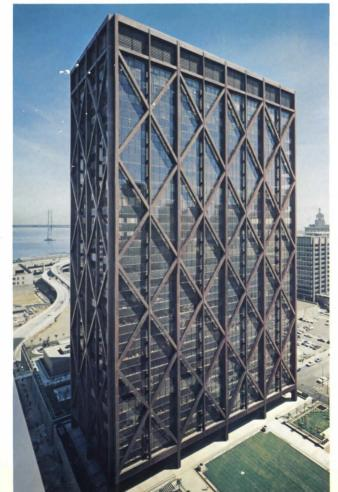
22-story Exchange National Bank Building, Tampa. Redesign in ASTM A572 steel (grades 50 and 55) saved \$45,000. Floor framing in office tower section is designed compositely with the slab. Architect: Harry A. MacEwen, A.I.A.
