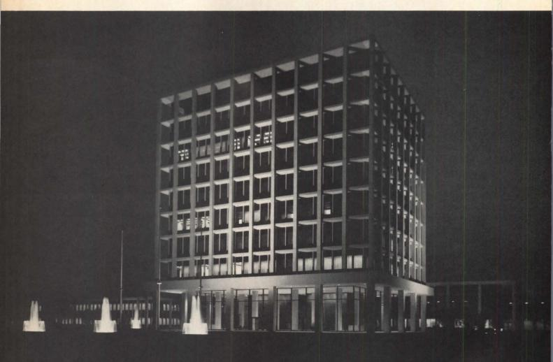
The face of Allstate Plaza is precast concrete panels of Indiana limestone aggregate. Sandblasting creates an interesting texture compatible with the rural surrounds. All precast and cast-in-place concrete contained PozzoLITH admixture.
