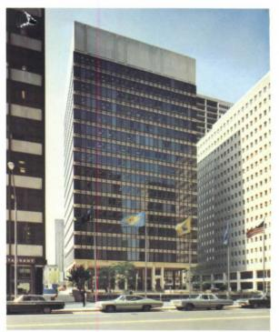
21-story IBM Building, Philadelphia (15 glass-enclosed office floors). Offset service core (not shown) serves as the backbone and steel framing serves as the rib cage to provide unusual openness and flexibility of space. Corrugated steel underfloors contain built-in channels for telephone and electrical wires. Architect: Vincent G. Kling, FAIA.
