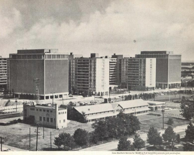
Ceco Steelform Service for 790,000 sq ft of monolithic concrete joist construction 12,700 tons of Ceco-fabricated Reinforcing Steel 480,000 sq ft of Cecocolor Anodized Aluminum Windows and Curtainwalls
