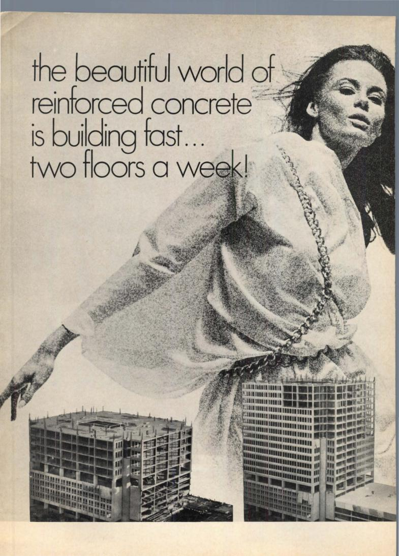
That's right. Philadelphia's newest office complex climbed that fast. It's the thirty-two floor, Industrial Valley Bank Building. Cast in versatile, economical reinforced concrete. With slim columns. On 30' spacings. Offering approximately 30,000 sq. ft. of ultra-flexible office space per floor. Exterior panels are dramatically sculptured reinforced steel precast sections that run 30' wide and a full story in height.
