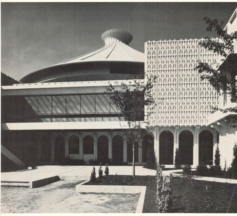
Quality concrete and fine craftsmanship combine to create the well-defined bas relief on the precast wall panels and the graceful molding above the corner vestibule.
