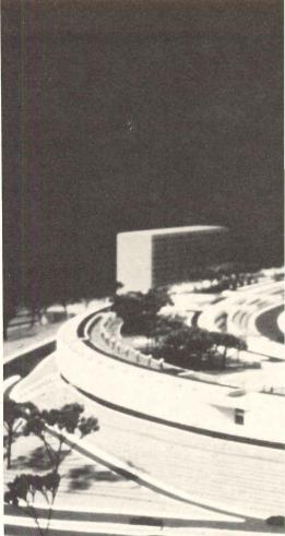
low. The bottom edge of the wall "floats" four feet above ground level, integrating the building with its site and visually separating it by the shadow that the light will cast in the void.
