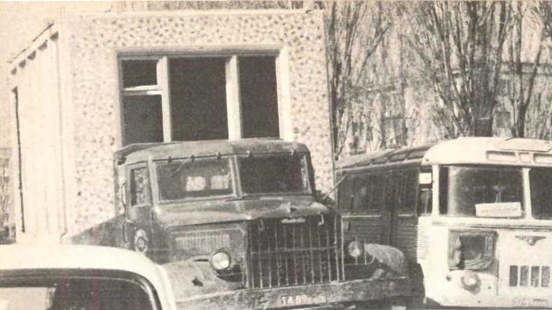
A prefabricated concrete-box being trucked to its site. Boxes such as these are just now going into mass production.
