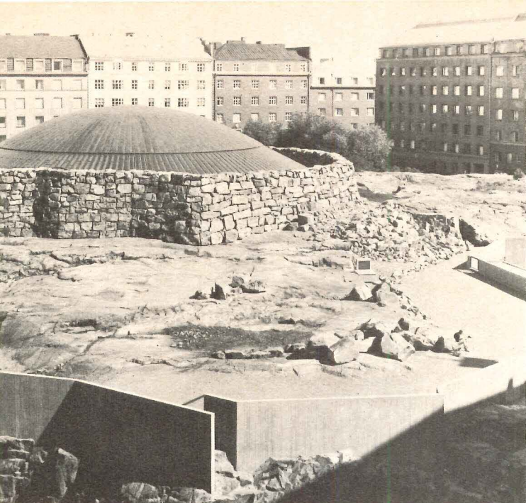
The plan shows how the church's interior was hollowed out of the solid granite outcropping, leaving exposed, blasted granite walls, topped by a translucent dome.
