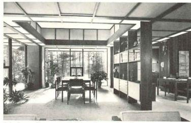
Interior walls are paneled in mahogany boards, plastered, or covered with carpet. Mineral acoustic tile covers all high ceiling surfaces, while low ceiling surfaces are acrylic/sand coated. The house and garage (photo, right) are separated some 50 ft to preserve existing trees and grade variation, and to establish a pleasant arrival space through which one walks enroute to the house.
