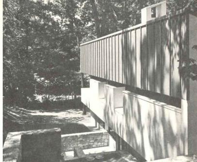
Wood floor joists cantilevered along the perimeter of the upper level support niches for storage space and provide a continuous chase around the exterior of the building for air supply ducts. Return ducts are housed in the attic space of the roof overhang.
