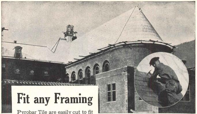
Pyrobar Tile are easily cut to fit around monitors, dormers and skylights. The light-weight, gypsum units also are erected quickly and economically on steep pitched roofs and curved surfaces.
