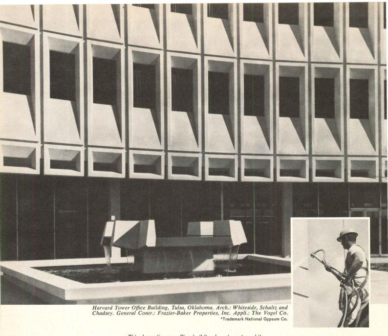
This dramatic new office building boasts a stay-white completely waterproofed finish. All surfaces (including the fountain) of block, precast concrete and Woodrock,\* inside and out, were sprayed with cement-base THOROSEAL PLASTER MIX plus ACRYL 60 which insures a tough bond. Time-and-money saving application finished Harvard Tower for occupancy without lingering labor costs.
