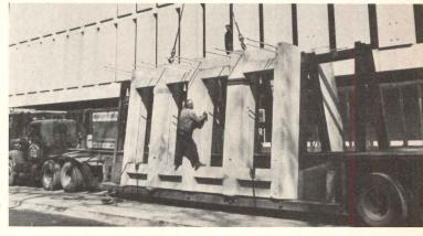
Precast load bearing units are 19'-11%" wide x 11' high. Average weight 12 tons. Spandrels are covered with black glass to accent vertical mullions.
