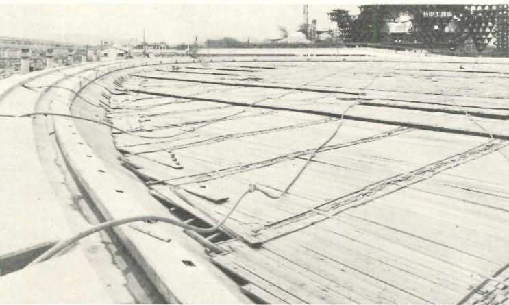
With falsework and cables in place, the roof was then laid out and laced to cables while work continued underneath.
