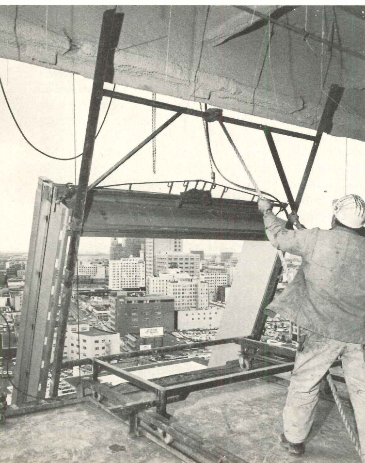
3. Assembled wall units are lowered into position from floor above.
