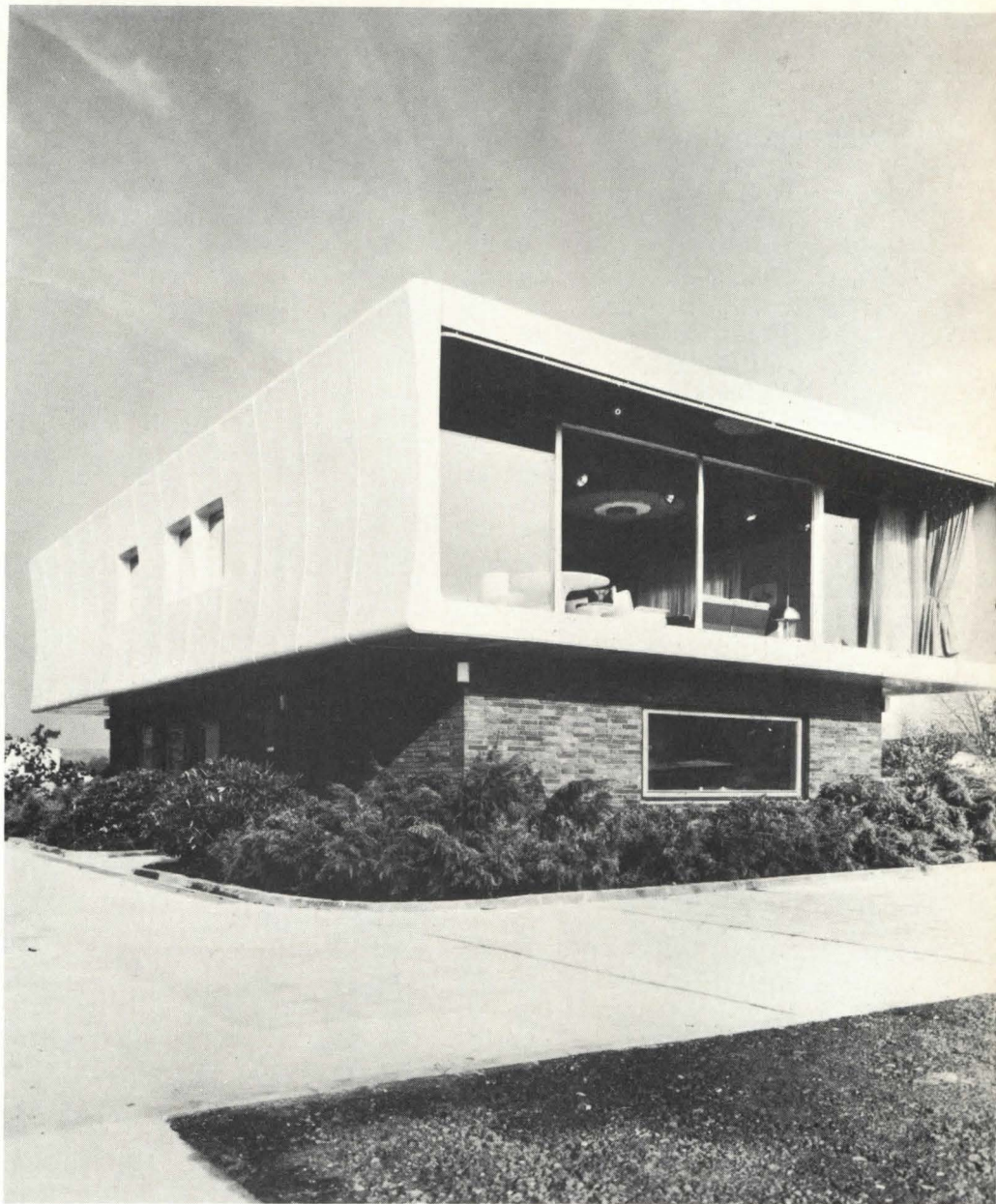
General view of German reinforced-plastics house incorporating molded glass fiber-reinforced plastic shells plus sandwiches for floor and interior surfaces.
