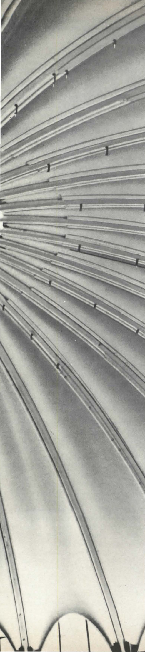
Hyperbolic paraboloid at Bangkok International Fair consists of glass fiber-reinforced plastics approximately 1/10-in. thick fastened to steel edge ribs. The roof is highly translucent. (Photo: courtesy United States Information Service)
