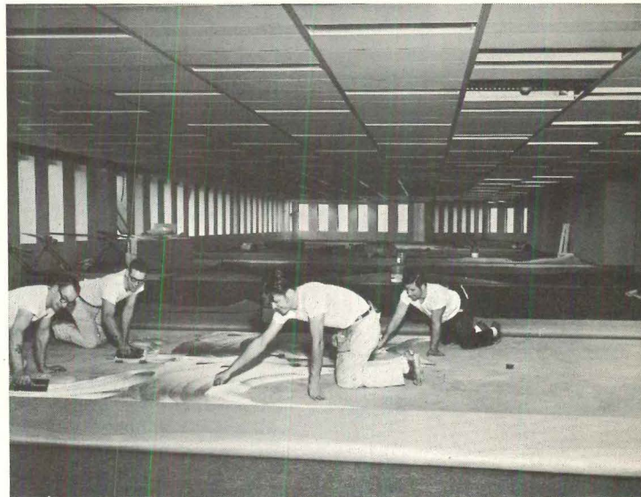
Installers applying adhesive to concrete sub-floor, for direct glue-down installation of double jute-backed carpets in new 64-floor U.S. Steel Building, Pittsburgh.
