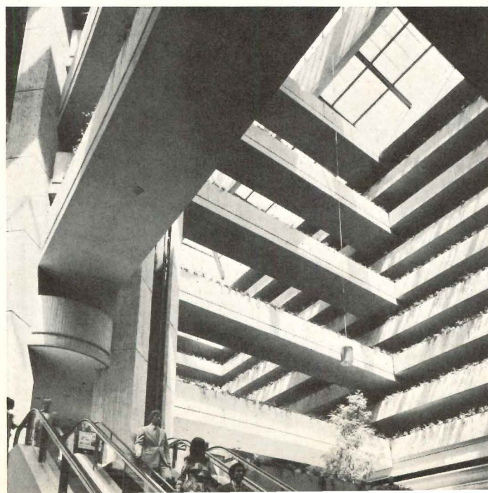
Escalators link convention facilities with main atrium lobby level. Concrete bridges link central elevator core to guest room balconies, changing direction at every other floor.
