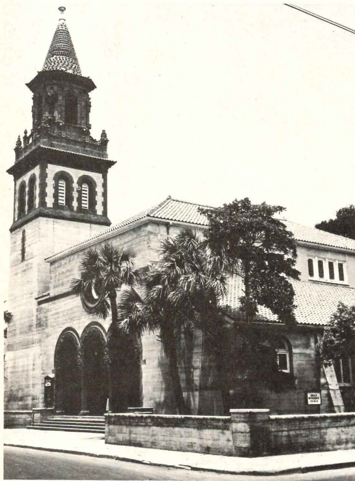
Grace Methodist-Episcopal Church is designed on a simple basilica plan. Use of mass concrete and king post timber trusses dates back to Roman era.
