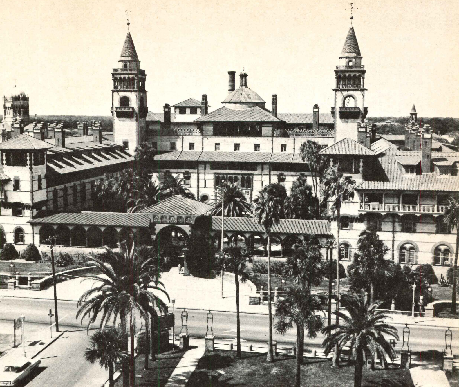
Ponce de Leon Hotel is now Flagler College. Architects Carrère and Hastings faced the concrete dome (left) with plaster.
