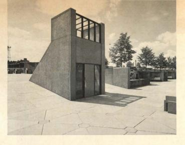
Entry to below-plaza parking garage (above). Open joint paving pattern allows rain to percolate through gravel fill to interior drains. All lighting is from concealed sources so that no fixtures clutter the plaza during daylight hours.
