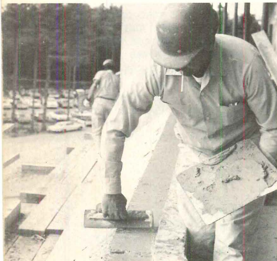
D. trowel coat to level
