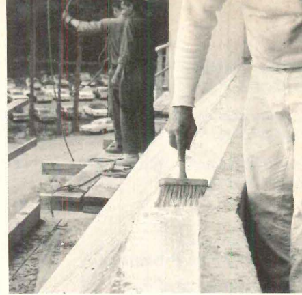
C. grout coat application
