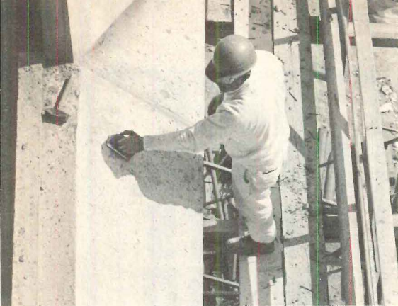
A. stoning rough concrete
