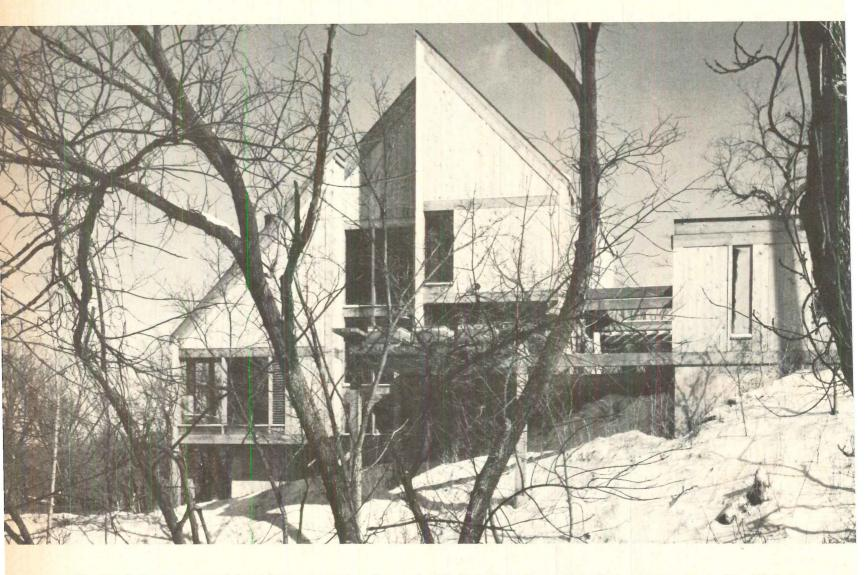
Meeting both site and spatial requirements, design of a wood house is based on a structural cage which defines the volumes that allow for changes in a couple's living patterns
