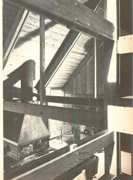
Structural cage is apparent outside the house as well as inside. Because of steeply sloping site conditions (above) and interlocking living spaces (right), a cage was selected to provide support for construction scaffolding as well as defining interior volumes. The nailed 2x4 roof deck spans between members in living areas.
