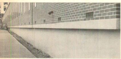
BASEMENTS – EXTERIORS: Based on the time-tested, cement-base THOROSEAL formula, but with coarser aggregates, THOROSEAL FOUNDATION COATING is specifically designed to protect and keep water out of exterior, below-grade surfaces, as well as beautify abovegrade foundation areas. Easily applied with standard or special Thoro coarse fiber brush.
