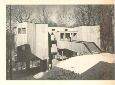
Standing high on wood pole foundations, the Bard College Modular Dormitories overlook a deeply wooded ravine, left. Sited just over the hill's crest, each of the seven units is entered by a bridge, above. Basic furniture units can be arranged as desired on predrilled walls.
