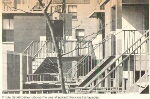
Photo detail (below) shows the use of scored block on the façades, the assymetrical rustication around the windows and the cantilevered block cornices at the roof. Photo above is taken across the bridge-like entrances to the four story units on Christopher Green.
