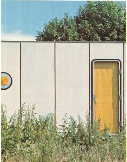
Guesthouse and carport of Rogers house, above, are framed with 3 steel bents; main house, beyond, is framed with 5 steel bents of same size. Bus doors and other openings, below, are neoprene-zipped into aluminum side sandwich panels. Front door, far left, is an 8' x 9' sliding glass panel.
