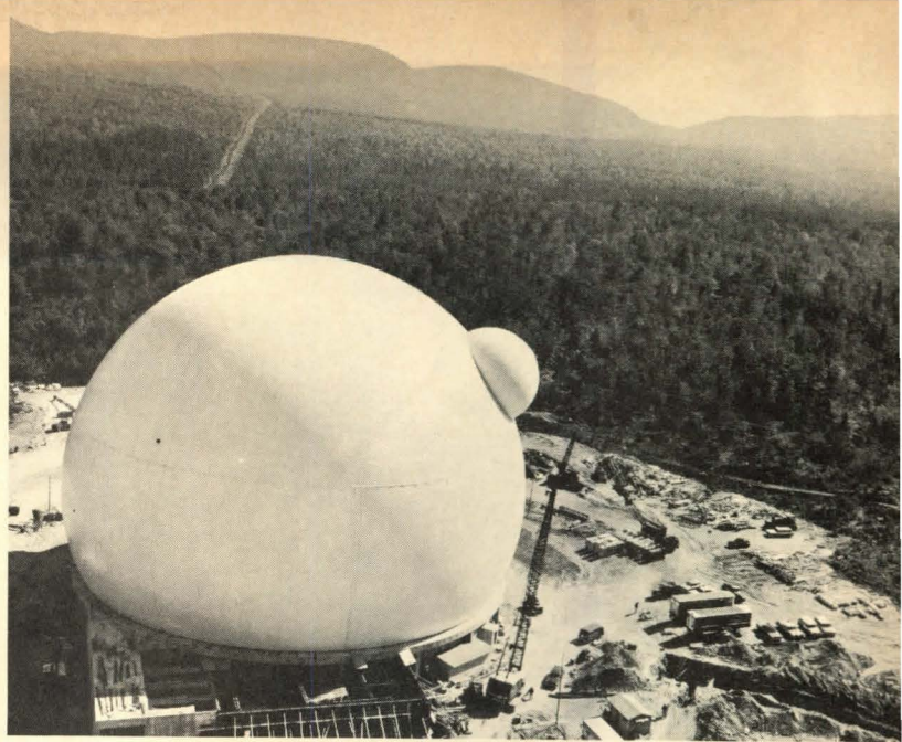
"Telstar" radome in Andover, Me, by Birdair Structures, Inc., is the largest example of a single-walled air structure to be built to date.
