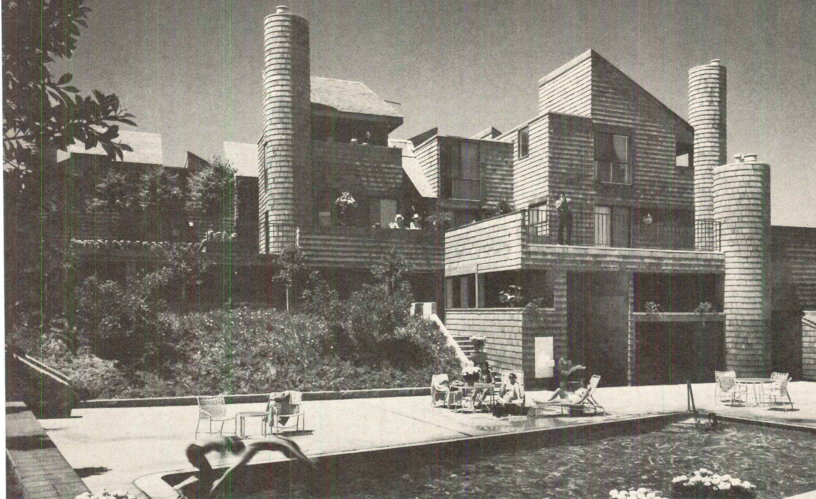
Seascape I, Solana Beach, California. Roofs: Certigrade shingles No. 1 Grade, 24" Royals. Walls: Certigrade shingles No. 1 Grade, 16" F... Architects: Oxley & Land...
