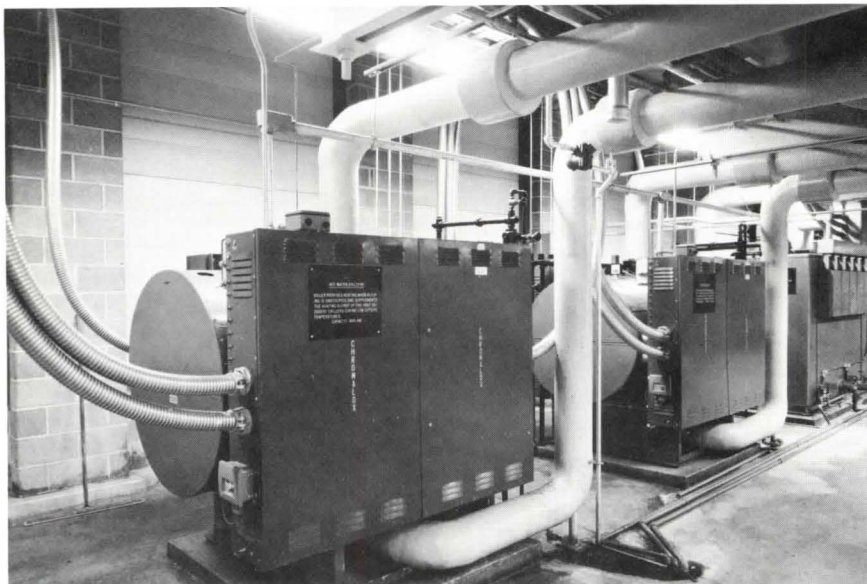
Twin 1800-kw electric boilers stand by to supplement recovered heat energy as needed.
