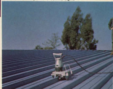
Closure tool "zips" the seams tight.
