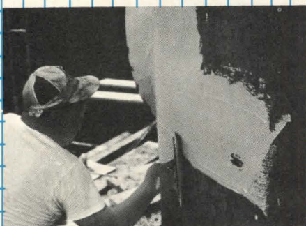
Applying finish coat April '72
