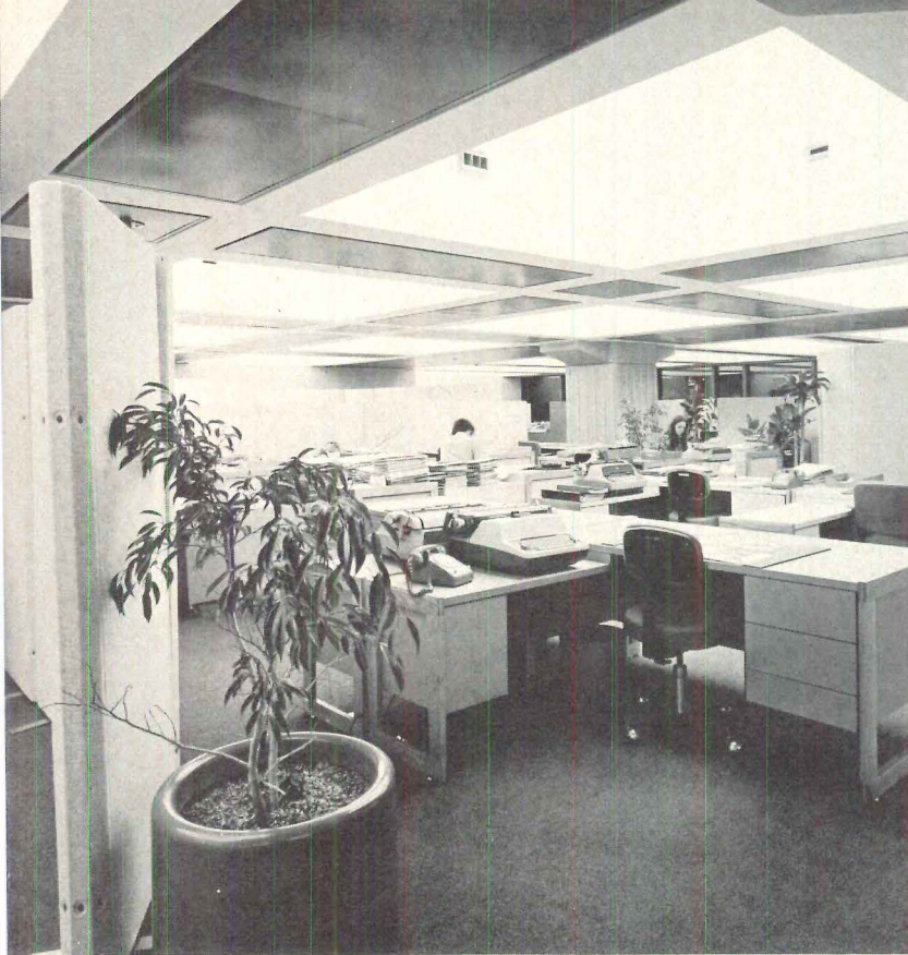
Integrated systems allow full use of office landscape (above). Tree column has holes for high velocity ducts, while those in the beams distribute air. Light sources are not visible.
