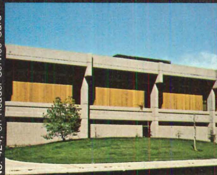
Ruf-Sawn redwood plywood combined with architectural concrete
