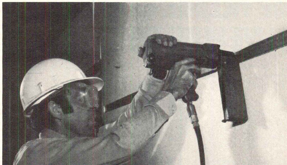
Nail through Foam to masonry.
