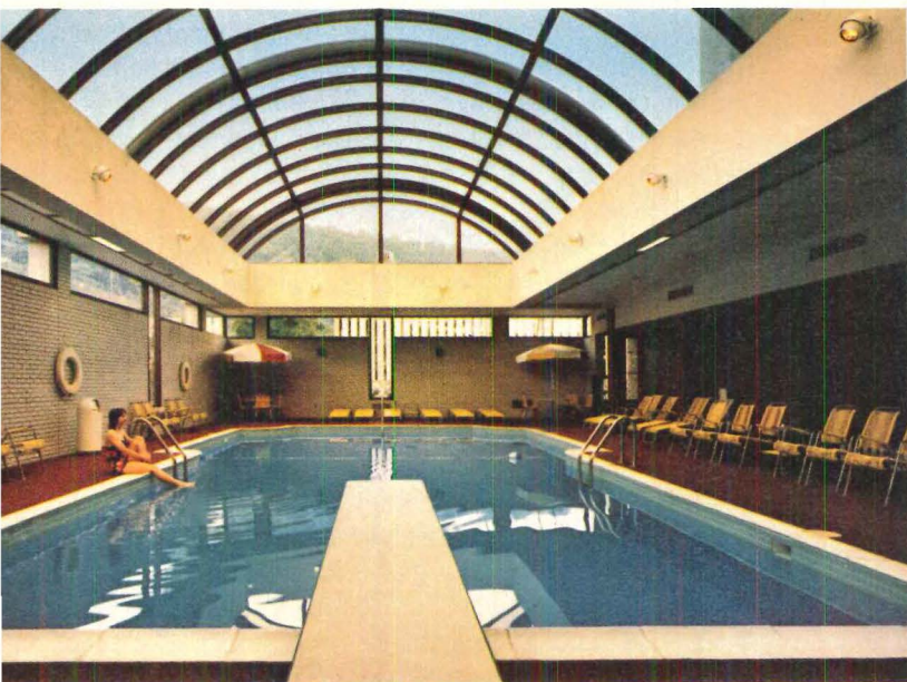
The clear span area in the first floor is over the pool. This enclosure measures 45 by 74 ft. The next major span is over the largest of the four meeting rooms, which measures 36 by 64 ft. This room can be evenly divided by a movable partition.
