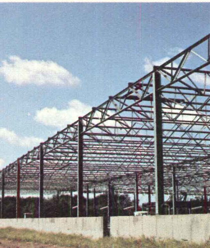
Joist girders have a simple span design. Which makes ponding calculations easier. And design time is shortened.
