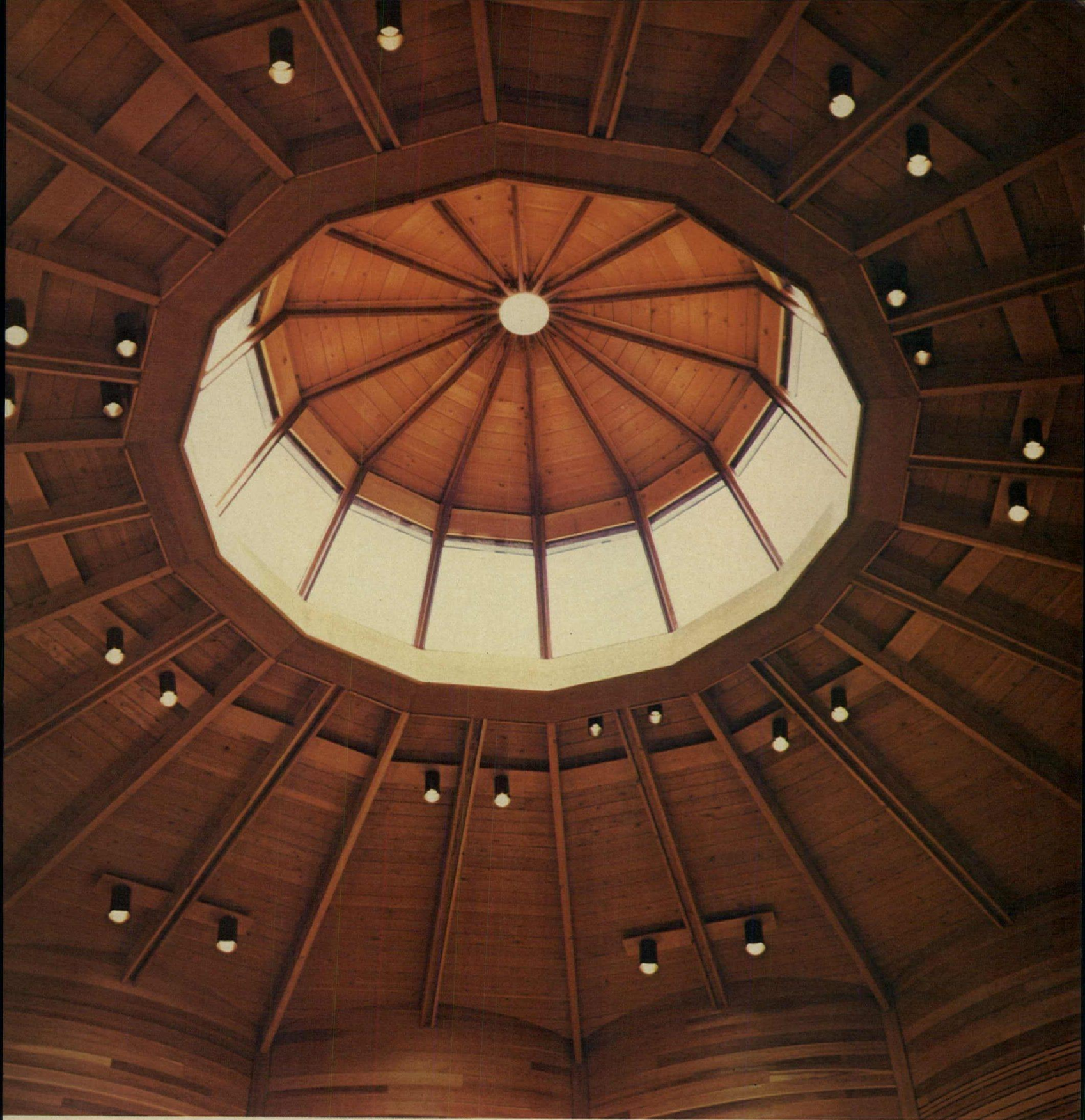
Mills College Chapel is composite design, concrete in compression, wood in tension.
