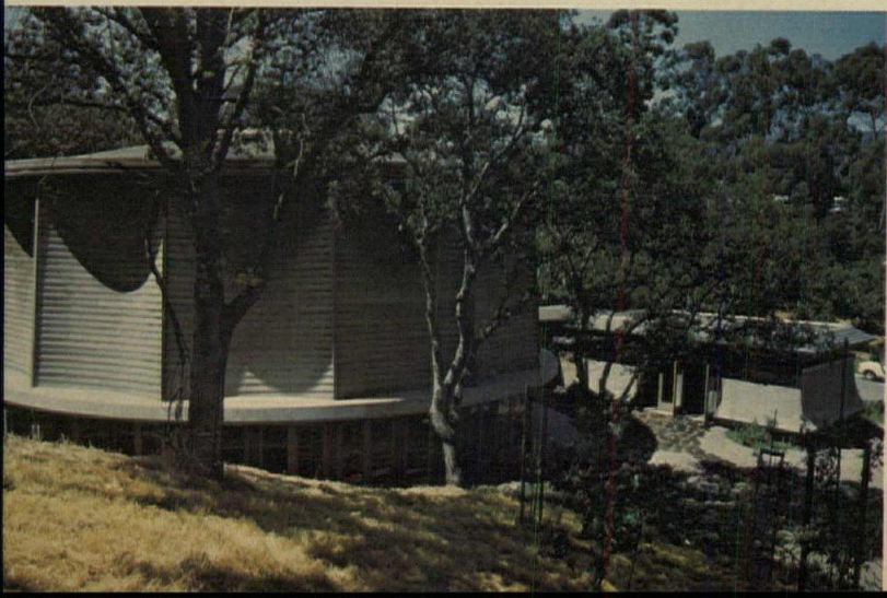
Mills College Chapel is composite design, concrete in compression, wood in tension.
