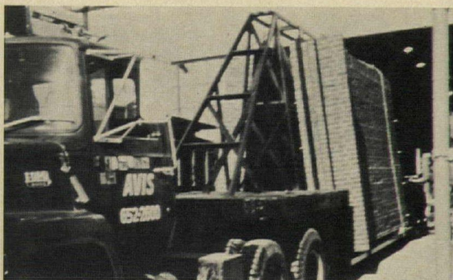
Pre-fabricated panels are easily loaded and shipped on flat-bed trucks to job-site.
