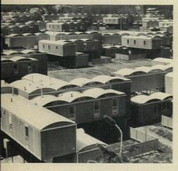
Modular fold-out units were used in Graphic Arts Center project, 1968 (above). Modules were suspended from trusses cantilevered from structural cores. Oriental Masonic Gardens was built in 1972 without foldout units (left). The Buffalo Waterfront proposal features foldouts that form cantilevered floors for three-level modular units; seen model (below and original diagram (bottom)
