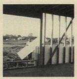
STYROFOAM TG insulation applied to the outside of a stud-frame commercial building. Installed in the same manner as conventional sheathing, STYROFOAM TG insulates as well as conventional sheathing and fibrous batts combined.
