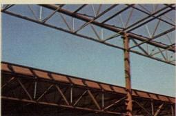
The light weight and simplicity of Vulcraft's steel joists and joist girders make erection fast and easy.
