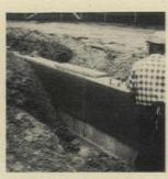
STYROFOAM insulation placed along the inner surface of a foundation in a perimeter application. Backfill pressure will not affect STYROFOAM.
