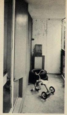
Large-scale furniture and rugs (above left) have trouble fitting economically scaled apartments. Balconies are well received, although some (above, right) function more as storage closets. Already paint has begun to peel, and rust form on metal dividers and trim. Tenants complain that balcony railing obscures the views.
