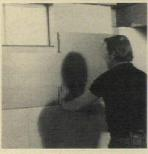
STYROFOAM brand insulation applied to the inside of a masonry wall with STYROFOAM brand mastic No. 11. Drywall will be applied directly to the STYROFOAM with the same mastic. After taping and spackling, decorative paneling can be applied with the same technique
