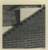
Cavity wall insulation with STYROFOAM. Because it is rigid board, STYROFOAM is easily installed in the cavity
