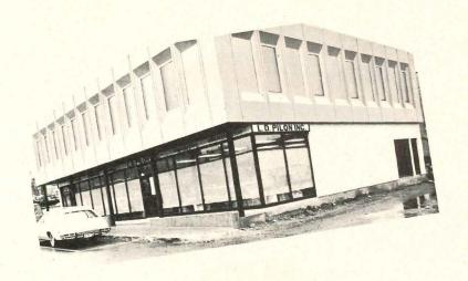
This new Molded Asbestos-Cement MAC70
