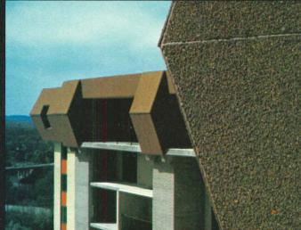
Prefinished stone aggregate, fire rated Aggreboard panels on steel studs installed on this luxurapartment building\* lowered costs considerably, reduces maintenance to minimum and enhances the exterior design with enduring color and texture
