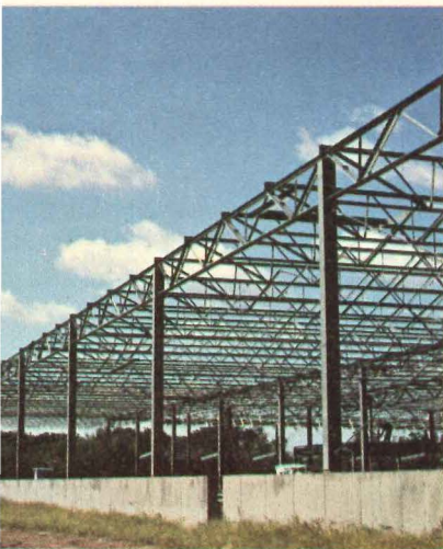
Joist girders have a simple span design. Which why ponding calculations are easier. And n time is shortened.
