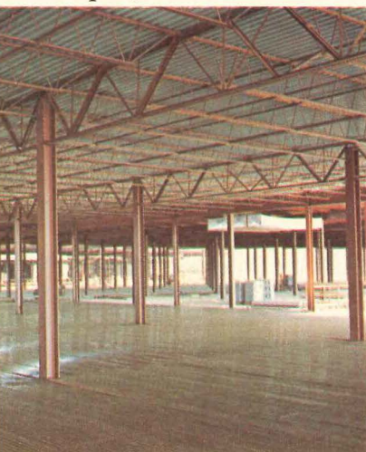
Joist girders need fewer foundations and Which means less work for you and larger for your clients.
