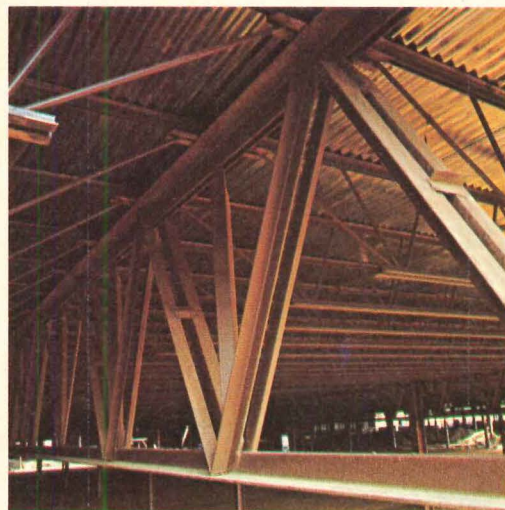
Joist girders have a modified Warren configuration using hot rolled double angle sections for top and bottom chords and single and double angle sections for web members. What that means is a high strength to weight ratio.
