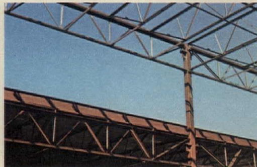
The light weight and simplicity of Vulcraft's steel joists and joist girders make erection fast and easy.
