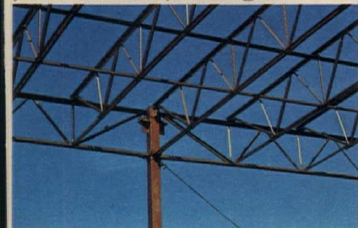
Vulcraft's steel joists and joist girders allow a standard five-foot module between connecting points.
