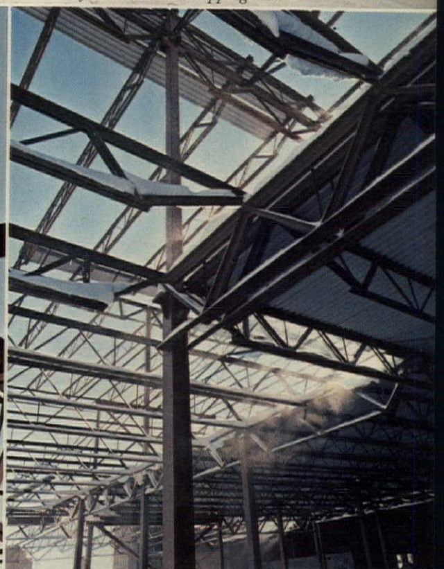
Joist girder design flexibility provided for a wide range of load support, from normal roof loads to heavy mechanical equipment loads.
