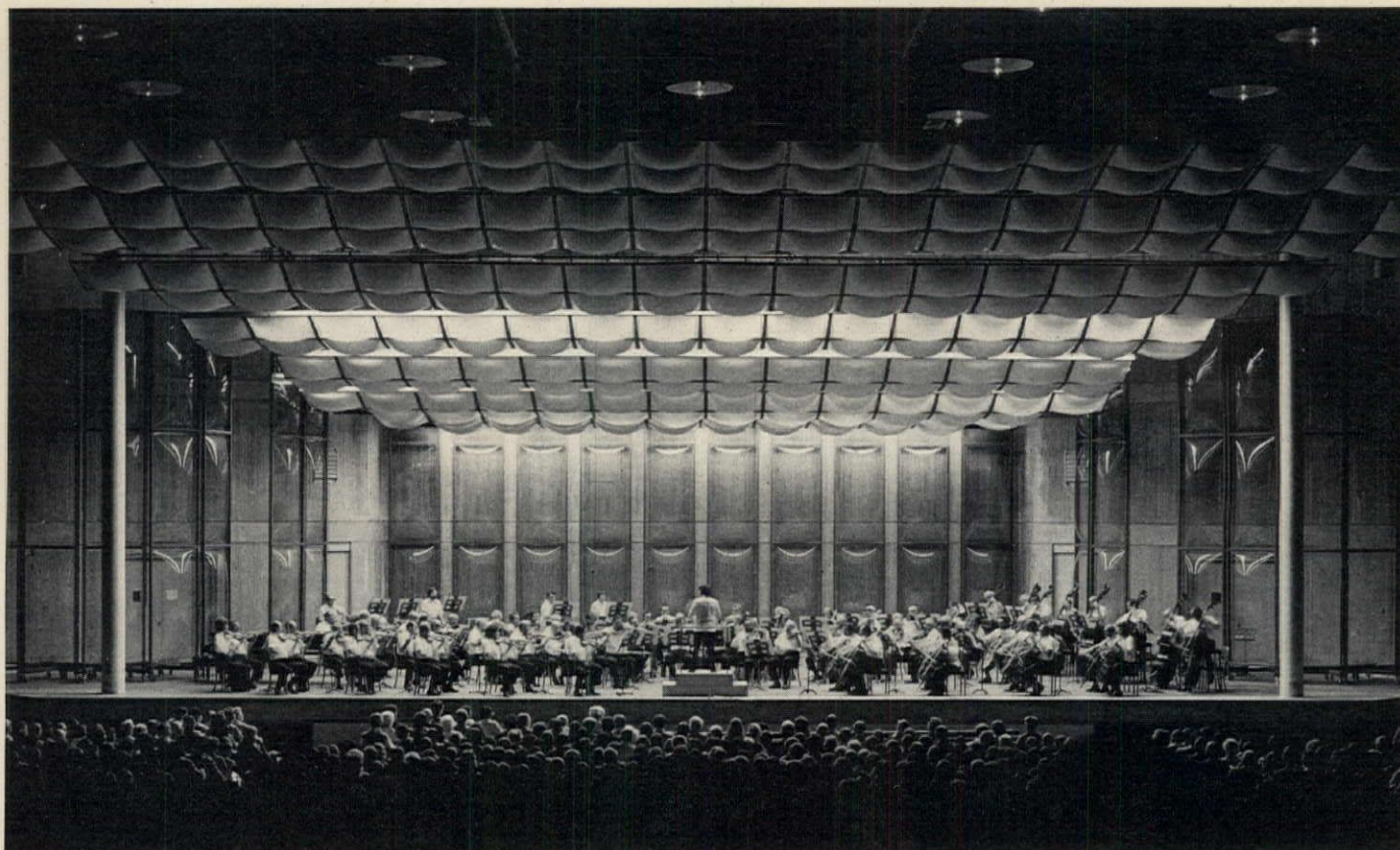
The concrete stage enclosure of Ravinia with acrylic reflector panels.
