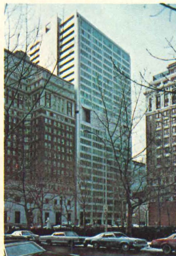
Penn Mutual's contemporary, the sleek, aluminum-clad INA Building, has recessed glazing except on north side.
