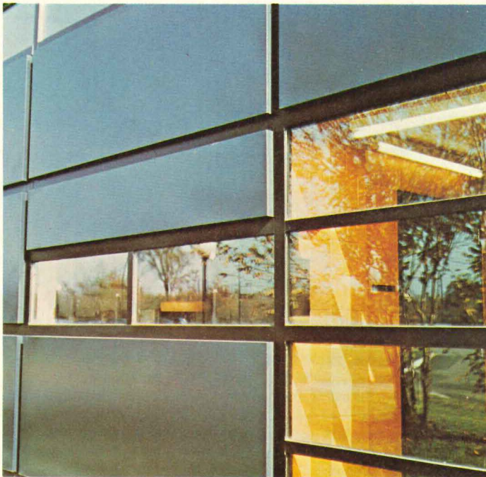
Bridge spans stream from core building (right) to skylit applied and general arts wing (above). Detail (below) of porcelain panel system.
