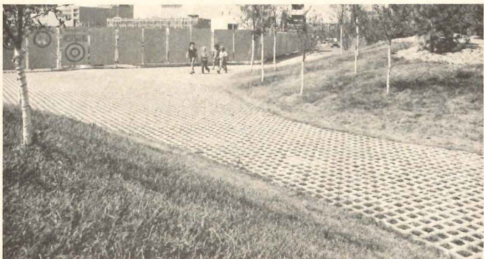
Grass can grow through concrete paving block with open pattern (above); interlocking block resists heavy loads.
