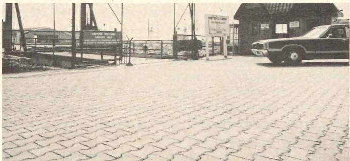
Grass can grow through concrete paving block with open pattern (above); interlocking block resists heavy loads.
