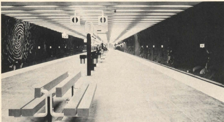
Suspended ceilings provide both lighting and acoustic absorption.
