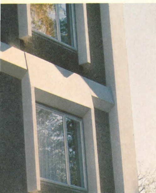
Cheesman Garden Apartments, Denver, Colorado Architect: Slater, Small & Spent; Denver Installation: Perma-Shield Casement operating and fixed units in precast frames
