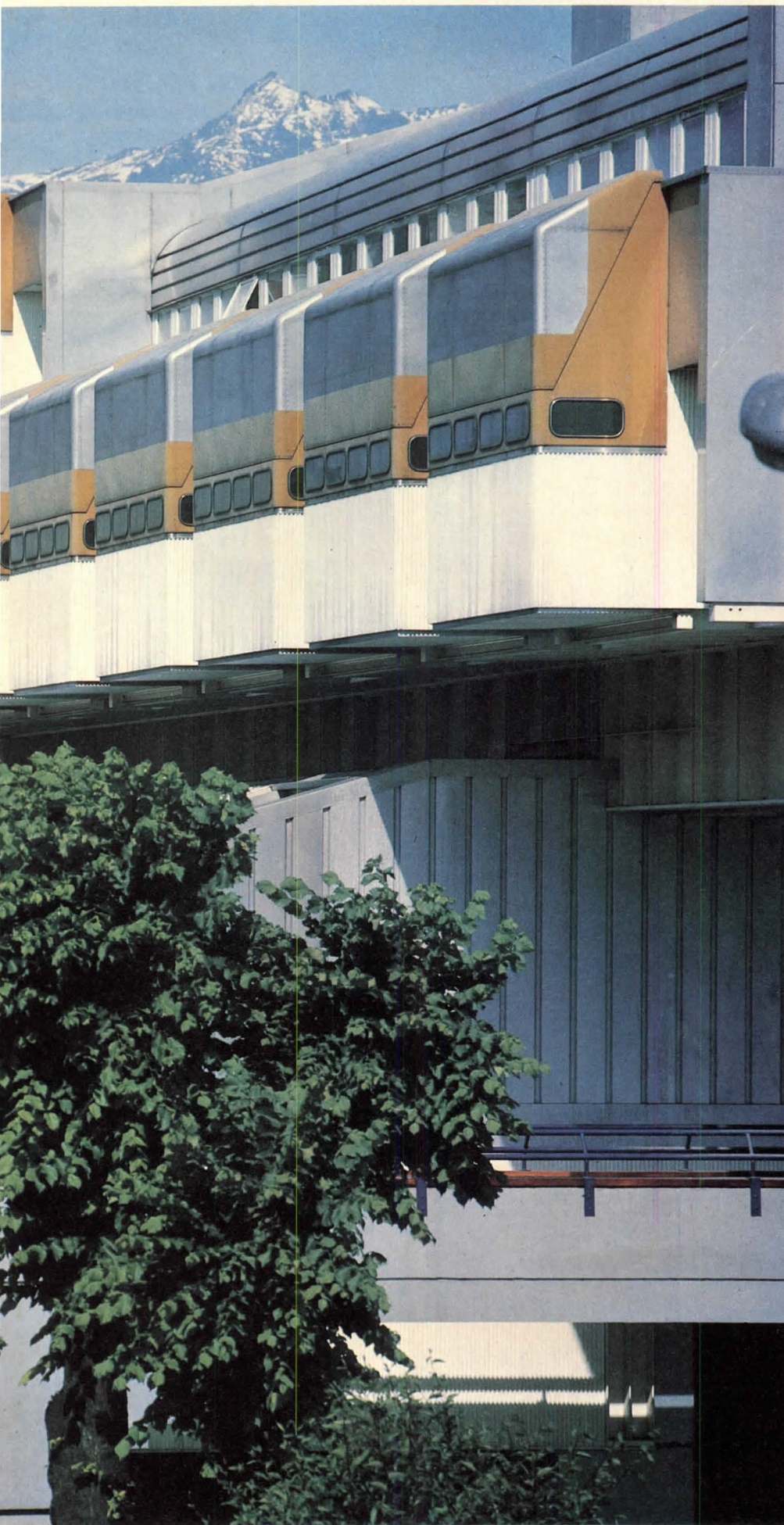
On the south side of Olivetti's compact-model megastructure (left) the prefabricated projections of the mini-apartments overlook a public park. On the north side, it confronts the staid, traditional fabric of Ivrea (top photo). Along the access street to the north (photo above) the new structure's massive concrete columns and aluminum-clad protrusions abut the weathered stucco of older neighbors.
