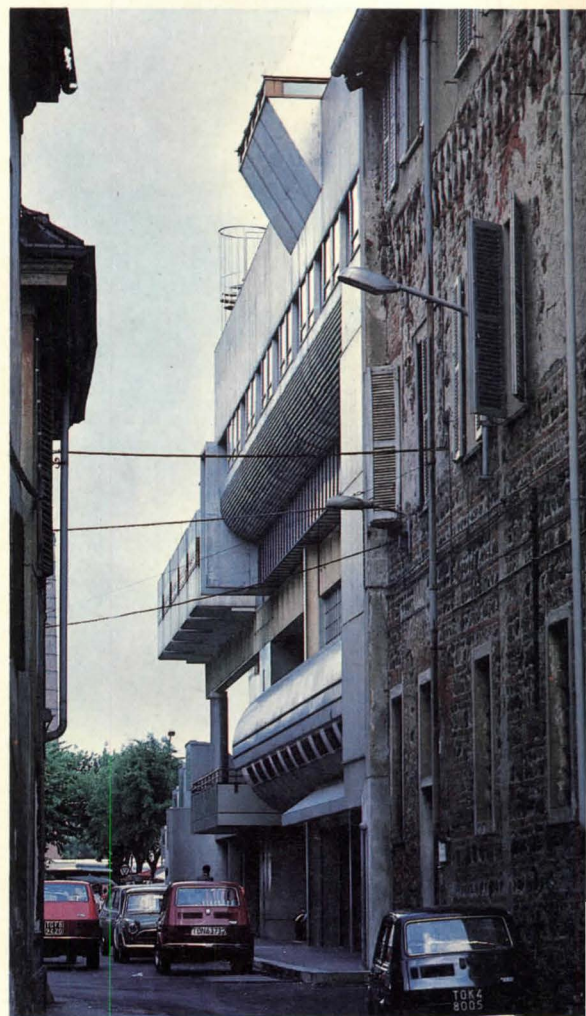
On the south side of Olivetti's compact-model megastructure (left) the prefabricated projections of the mini-apartments overlook a public park. On the north side, it confronts the staid, traditional fabric of Ivrea (top photo). Along the access street to the north (photo above) the new structure's massive concrete columns and aluminum-clad protrusions abut the weathered stucco of older neighbors.
