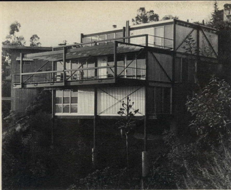
By using a modular coordination grid, the TEST house integrates a wide variety of preindustrialized components into a single, flexible building.
