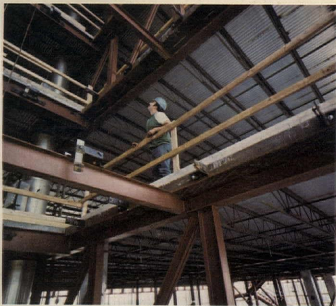
Interior view during construction shows large, column-free spaces. Typical bays measure 53 ft 6 in. by 22 ft. Bethlehem supplied 700 tons of structural steel for the project.
