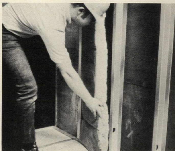
Two forms of wall insulation. Batt or blanket materials are available with a number of facings. Mineral fiber batts with kraft paper facings give effective fire and vapor protection (above, in steel stud wall). Fire and vapor barrier also are achieved by semi-rigid glass boards (below) also bar fire and vapor.
