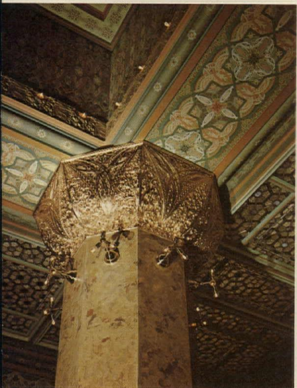
Scagliola on the columns survived in part; new artisans were found to recreate the artificial marble finish.
