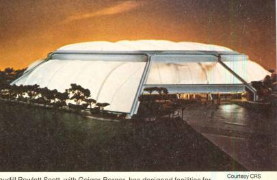
Caudill Rowlett Scott, with Geiger-Berger, has designed facilities for The University of Florida in Gainesville (above) and The University of South Florida (below). Both are air-supported, but the Gainesville job incorporates Teflon/fiberglass tensile structures on the perimeter.
