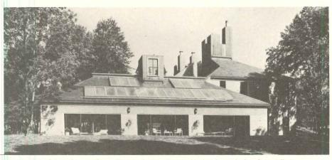
Pool pavilion (above) has solar collectors for heating and belvedere window for cooling. Living room (right) has indirect lighting, belvedere windows.
