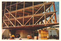
High-strength steel trusses enabled the architects to create a unique cantilevered design for this six-level bank and office building. Bethlehem supplied 340 tons of steel for the project.
