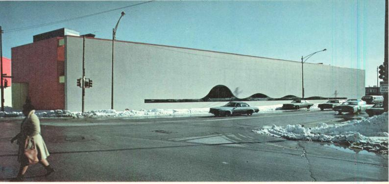
Poured concrete wall acts as a beam to span 165-ft-long butt-jointed window, elsewhere. Panels on exterior of building are baked enamel.
