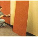
Panels are sound-absorbing eral-fiber board covered with crylic fabric. Grooved edges ck into concealed aluminum splines, make installation an
