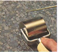
Seams are chemically welded to provide a continuous surface that resists penetration of dirt and moisture.
