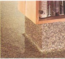
Brigantine can be coved where the floor meets the wall to help eliminate places where dirt can hide.
