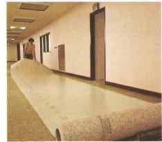
Rolls 6' wide and up to 90' long keep seams to a minimum, provide an almost monolithic look.
