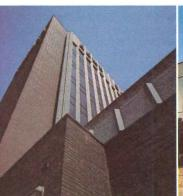
High 110' structure enjoys substantial look of masonry but without the weight of a reinforced masonry wall.
