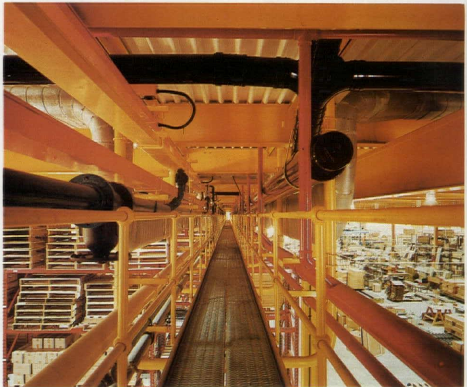
Internal flexibility is important in the open-plan factory; all main services are reached from a centrally located overhead catwalk (above); and toilet stalls (below and left) are portable.
