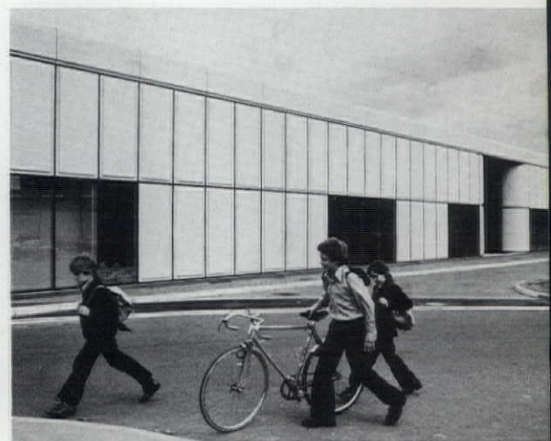
Like Herman Miller's Action Office furniture, which is produced at this plant, the building also uses cream-colored fiberglass panels and curved corners. South side faces River Avon (left); main entrance is at the west (above), and parking is at the rear, north side (below).
