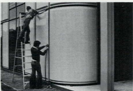
External cladding system uses fiberglass panels (above, below), glazed or louvered panels (top).
