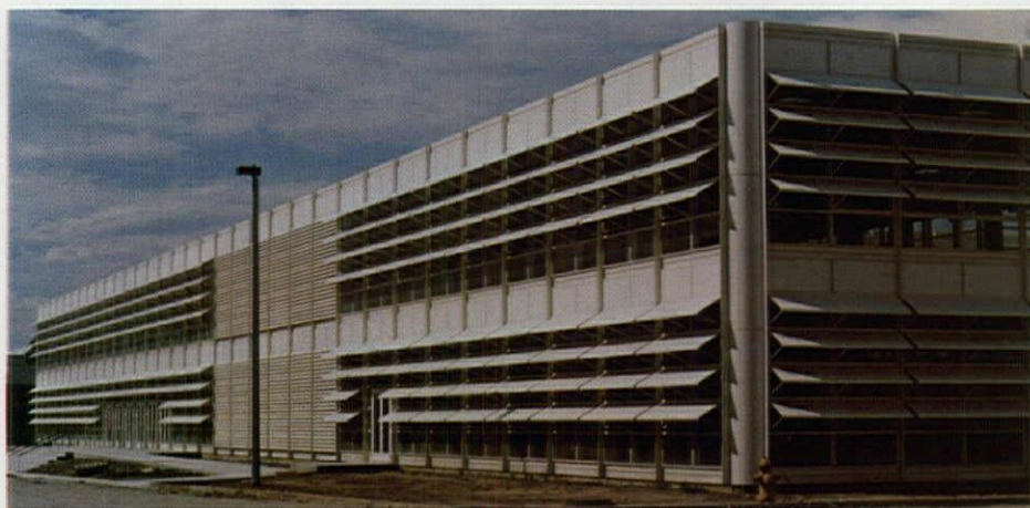
Sunscreens protect west, entry side and south side (above), but not east office side (below).
