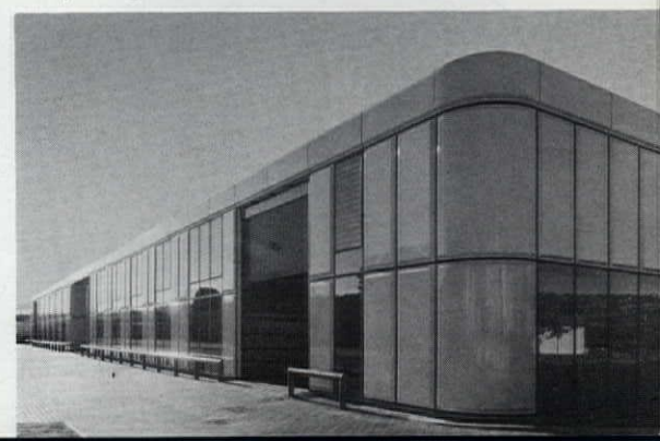
Like Herman Miller's Action Office furniture, which is produced at this plant, the building also uses cream-colored fiberglass panels and curved corners. South side faces River Avon (left); main entrance is at the west (above), and parking is at the rear, north side (below).
