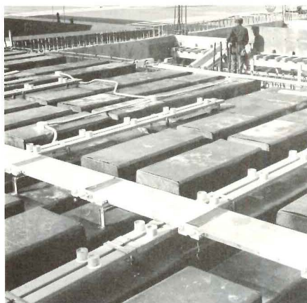
Trenchduct and insert system in concrete slab.
