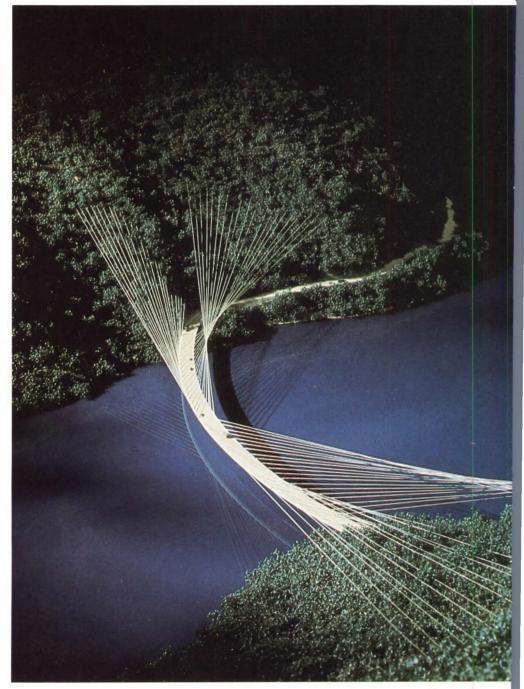
crete box girder solutions exist for the curved deck. Either solution would be constructed by cantilevering from each side abutment towards the center, controlling bending moments during construction with horizontal erection cables. Bridge geometry accommodates repetition of elements and/or formwork. An excellent explanation of the workings of this bridge can be found in ASTM Reprint 3305 written by T.Y. Lin and D. Allan Firmage entitled: *The Design of the Ruck-A-Chucky Bridge*.
