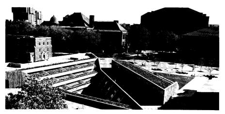
A good example: Williamson Hall on the Minneapolis Campus of the University of Minnesota. It's a site-cast reinforced concrete structure, 95% of which is below grade level.
