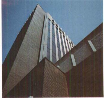
Mini-Brick simplified engineering and shortened construction schedule in 110' steel structure as construction moved at its own pace, not tied to the masonry.
