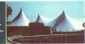
In addition to low construction costs, fabric structures coated with TEFLON offer easy and economical maintenance. The coated fabric resists sunlight, dirt and aging, and rain helps keep it clean because of the non-stick surface of TEFLON.
