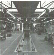
airy atmosphere; on either side of the mechanics' pits, skylit roof sections provide daylight for work areas.
