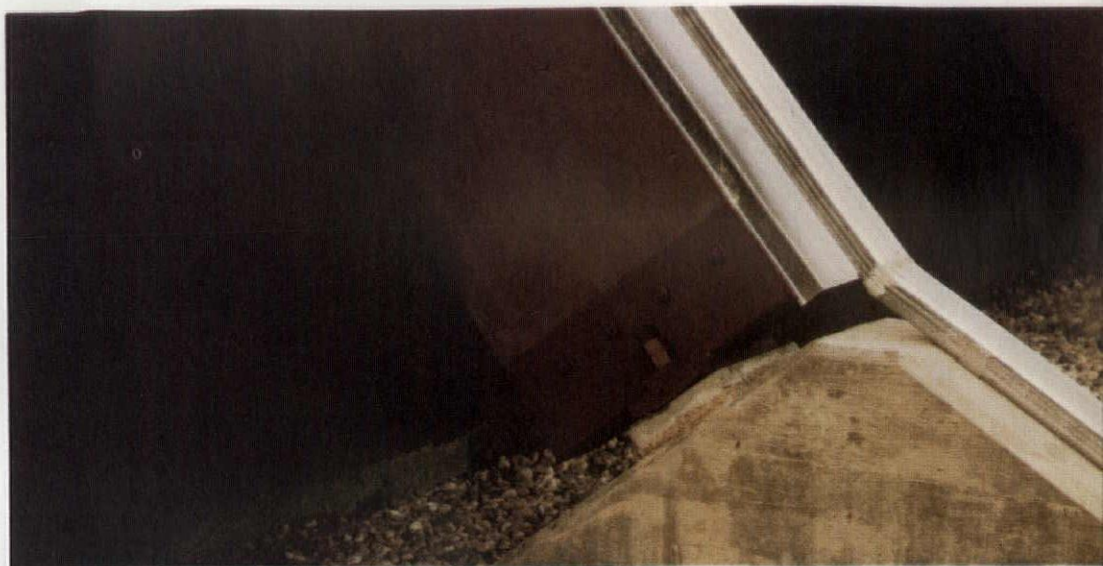
Wood which comes in contact with moisture must be detailed to shed the moisture either directly or through evaporation. Bad design can cause decay (above and below) and rot.
