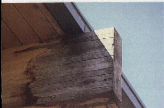
An overhang often makes very good engineering sense when using glue-laminated beams. Care must be taken, however, to limit the contact which the overhang has with the weather. The end grain of all wooden beams is susceptible to moisture penetration. One answer is to angle the cantilever ends (right). Bushes and plantings which are watered daily should be kept away from the exposed bases of wood arches (far right). All photos: AITC
