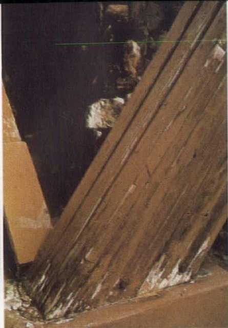
Wood which comes in contact with moisture must be detailed to shed the moisture either directly or through evaporation. Bad design can cause decay (above and below) and rot.
