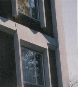
Installation: Perma-Shield casement operating and fixed units in precast frames
