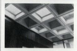
Insul-Art™ acoustical products, with cores of glass fiber materials for sound control, include wall panels and ceilings suitable for offices, schools, auditoriums, gymnasiums, and other commercial buildings. Wall panels ranging up to 5′ x 12′ x 2″ thick are available straight or curved, with square-cut, beveled, or radiused edges, and square-cut or radiused corners. Ceilings include coffers, lay-in panels, and duct-type tubes. Company's standard fabrics [Products continued on page 240]
