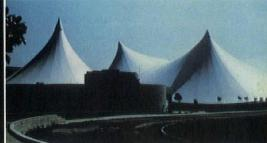
In addition to low construction costs, fabric structures coated with TEFLON offer easy and economical maintenance. The coated fabric resists sunlight, dirt and aging, and rain helps keep it clean because of the non-stick surface of TEFLON.
