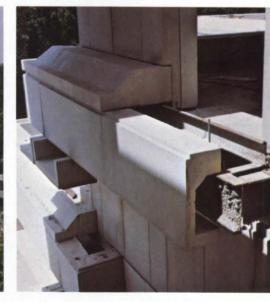
Some 1,100 tons of A36 steel were used in the construction of the West Headquarters Building. The steel frame simplified the many connections required for the precast concrete exterior, as well as installation of the mechanical and electrical systems. The 162,000-sq-ft office building, located on a hillside across an entrance plaza from the original headquarters building, provides modular office space for 650 employees.
