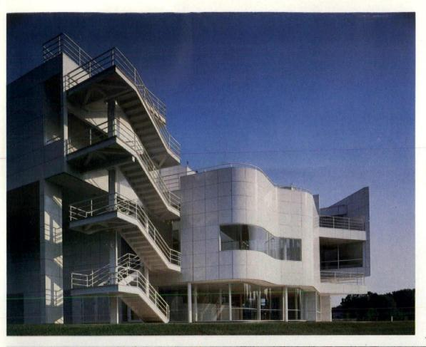
Routes of egress from the rooftop and upper-level terraces take visitors through punctured planes and screen walls and past curved and screen wans and past curved surfaces, most of which are cov-ered by the 2'-6" porcelain-enameled panels. One wall at a five-degree angle is sheathed in panels five feet square.
