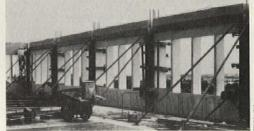
PRECAST CONCRETE LOAD BEARING PANELS
