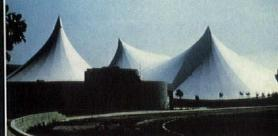
In addition to low construction costs, fabric structures coated with TEFLON offer easy and economical maintenance. The coated fabric resists sunlight, dirt and aging, and rain helps keep it clean because of the non-stick surface of TEFLON.
