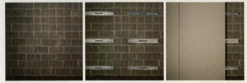
By eliminating common studs and batt insulation, the Thermawall Insulation System reduces installation costs dramatically, going from metal channels to finished drywall in one step.
