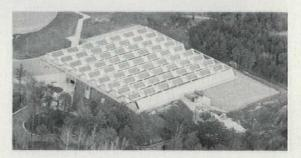
To reduce heat loss and gain, the building is set four feet below grade, with the soil removed for excavation forming a berm of insulation around all but the building's north side, where double bronzed glazing is used to give views to the lake and woods beyond.
