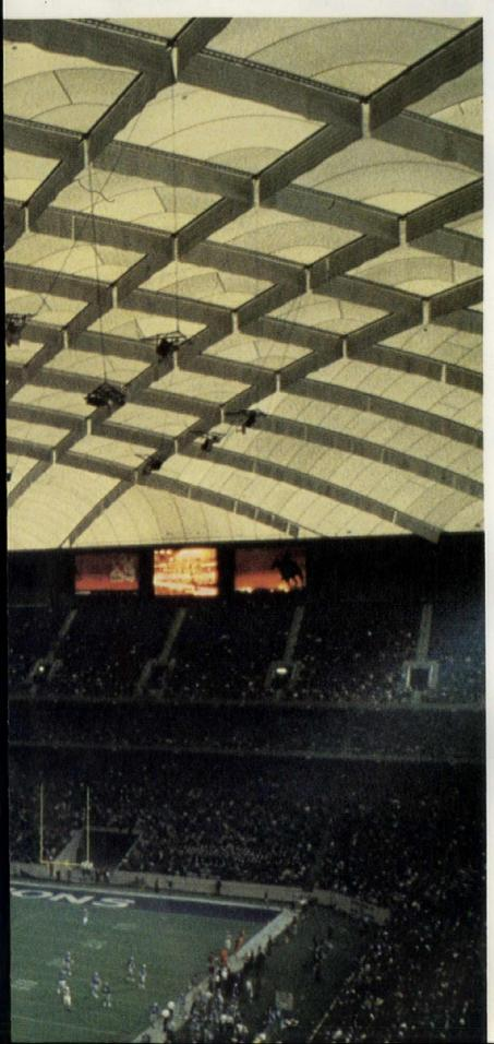
An air-supported dome of lightweight Fiberglas® coated with DuPont TEFLON® fluorocarbon resin completely roofs Pontiac Silverdome, home of the Detroit Lions, Detroit Pistons and Detroit Express. The 10-acre area is the largest permanent structure roofed with architectural fabric to date—and the stadium cost far less to build than comparable stadiums using other dome approaches.
