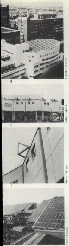
5 Solar collectors cover the roof of a bank in Japan. 6, 7 In the Naoshima Citizen Gymnasium, Architect Kazuhiro Ishii and solar consultant Saburo Takama collaborated to combine solar water heating and daylight control. 8 Solar heating, cooling, and pool water heating are accomplished in the Doho Park Gymnasium. The architects Masato Ohtaka Associates were assisted by solar consultant Saburo Takama.
