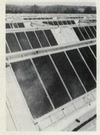
The sawtooth roof at the Shenandoah Recreation Center supports both solar collectors and reflectors at their respective optimal angles of 45 and 36 degrees (above); further advantages are gained through berming and burying the 58,000-sq-ft structure.
