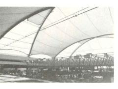
heerfill® architectural fabric berglass coated with Teflon® is used in ranslucent roofing systems. The white, 5 percent reflective exterior surface educes heat gain from the sun while llowing in enough light to cut daytime ghting needs. The result is a reduction f heat buildup and consequent lowerng of air-conditioning load. According o the manufacturer, the material is lassed as noncombustible by all model ode agencies. Chemical Fabrics Corp., irdair Structures Division.
