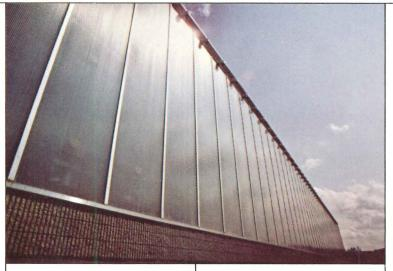
Two basic components of the solar system are a 12-inch concrete block wall and EXOLITE double skinned acrylic sheet as the glazing material. The EXOLITE sheet is several inches from the concrete wall, providing a chamber into which cooler air enters through openings in the bottom of the wall. Air is returned to the room through openings at the top after being heated, as it flows over the surface of the warm wall.
