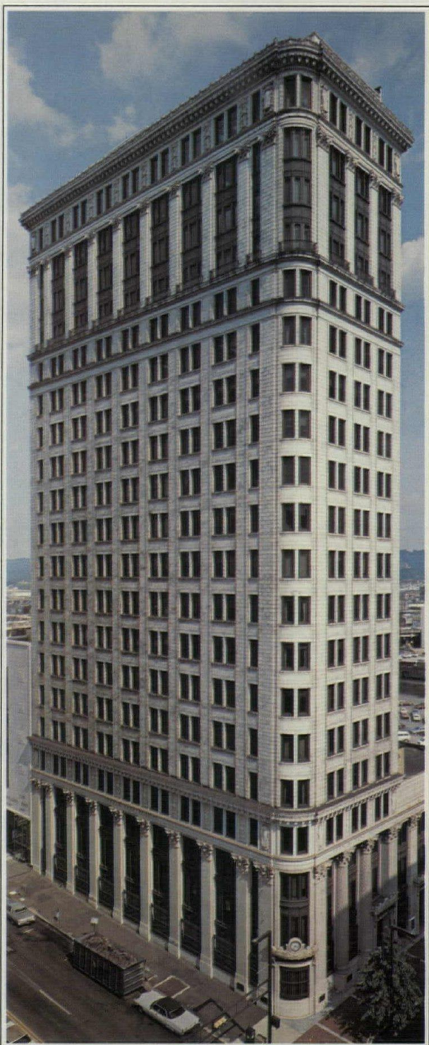
John A. Hand Branch Office, First National Bank of Birmingham, Alabama's Largest Bank. Brice Building Co., Inc., General Contractors.
