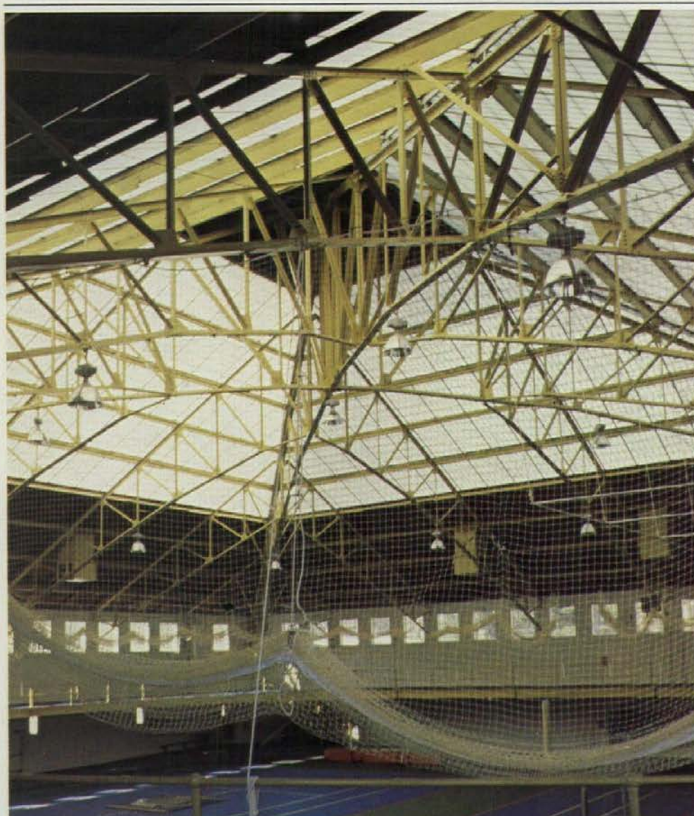
Skyroof Retrofit Johnson Holvett Di Nisco & Associates, Architects
