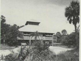
The house is next to a tidal estuary, and it is raised high on wooden poles set deeply into the ground. Clerestory windows in the belvedere induce ventilation. The tin roof with wide overhangs reflects heat and shades windows, and also permits windows to stay open during rainstorms. Entry at east side (right) leads directly into "dog trot" living area.
