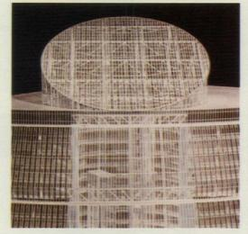
massive skylight. These features will take advantage of enough passive solar heating and natural light to reduce energy usage to nearly one-half the level consumed by most conventional office buildings. Since artificial lighting generally consumes 40% of a building's energy load, any heat lost through the glass walls will be more than offset by the cost reduction achieved through natural lighting. These factors, the architects and
