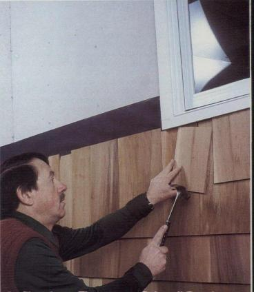
As Sheathing, Thermasote Sidewall Panels Provide A Tough, Structural Nail Base Insulating Sheathing For Finished Siding.
