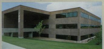
Plaza 7000 office building, Denver, Colorado. Panelized system used. Desert Brown Mini-Brick was mounted on panels within the building, then the panels hung from the inside. No scaffolding. No downtime from weather. Estimated savings: \$1 per sq. ft. compared with 4" brick for the 18,000 sq. ft. facing. Developer: Orr Associates, Inc. / Tile contractor: Hi-Lo Tile / Distributor: Brick, Inc.
