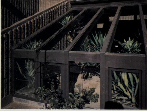
Above & below. The "greenhouse" provides an additional heat sink which employs the floor and concrete masonry walls for heat storage. The diagram below shows the orientation of the building to low Winter and high
