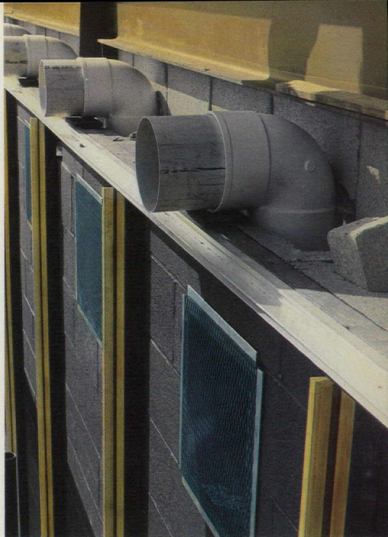
A construction photo showing the venting ports which exhaust trapped solar heating to the outside in Summer. The grilles shown, transfer heat to the inside during Winter. Diagram at left shows how the system operates.
