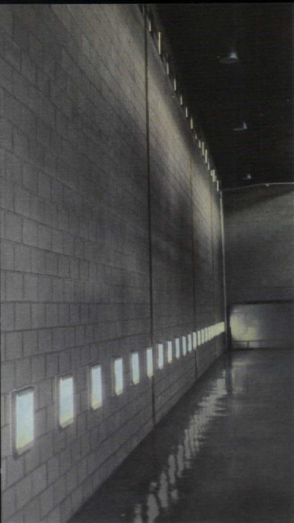
Standard 12x8x16" concrete masonry units, grouted solid and painted black on the exterior, are employed in the Trombe wall.
